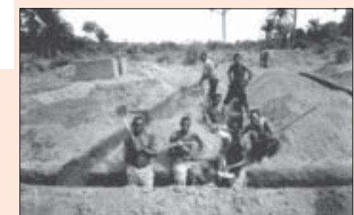
Digging the foundation of the guest house in Baguga.
